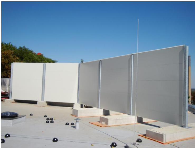
Fig. 4. Mobile noise barrier with openings [10,17].
