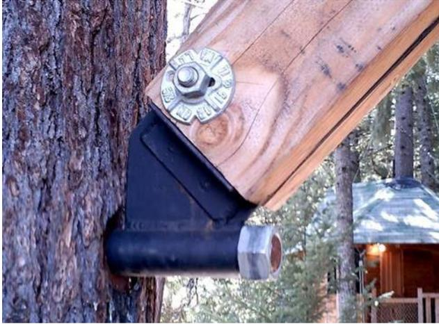
**Figure 1.** Mechanical anchoring to the tree.
