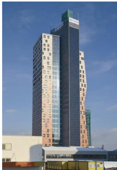
Figure 1. High-rise building with the PV façade
