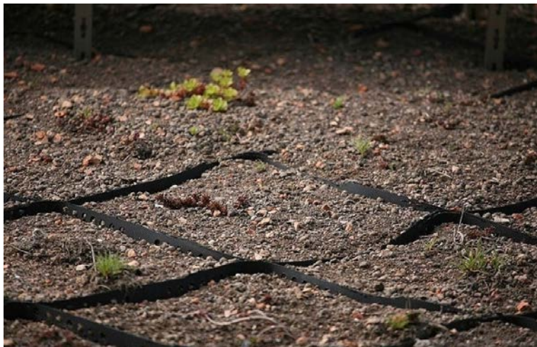
Figure 3.: Example of unequal consolidation of the substrate and geocell.
