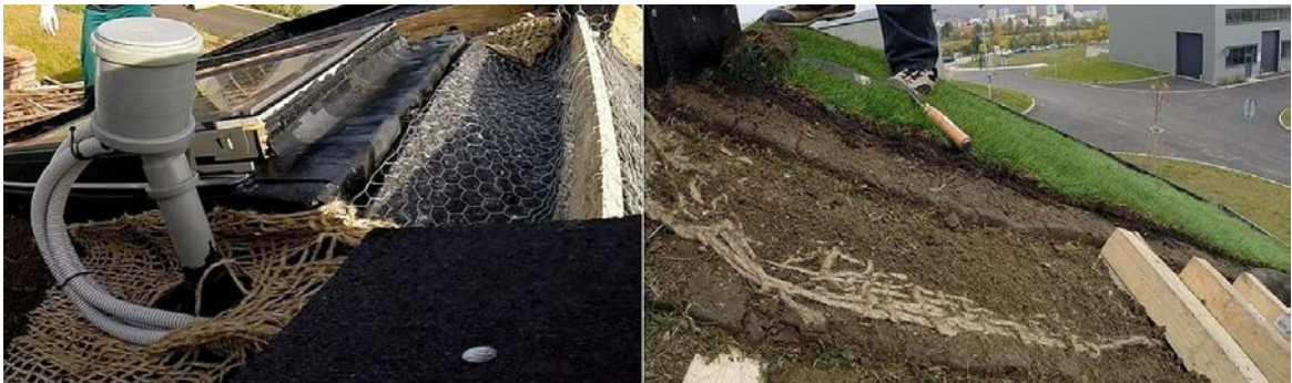
Figure 4.: Anti-sliding system of the biodiverse (left) and of the Icelandic green roof (right).
