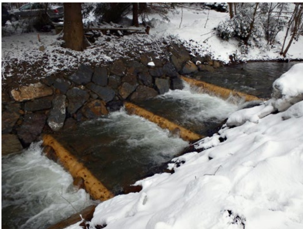
Fig. 101 Cascade – the high weir divided into three steps
