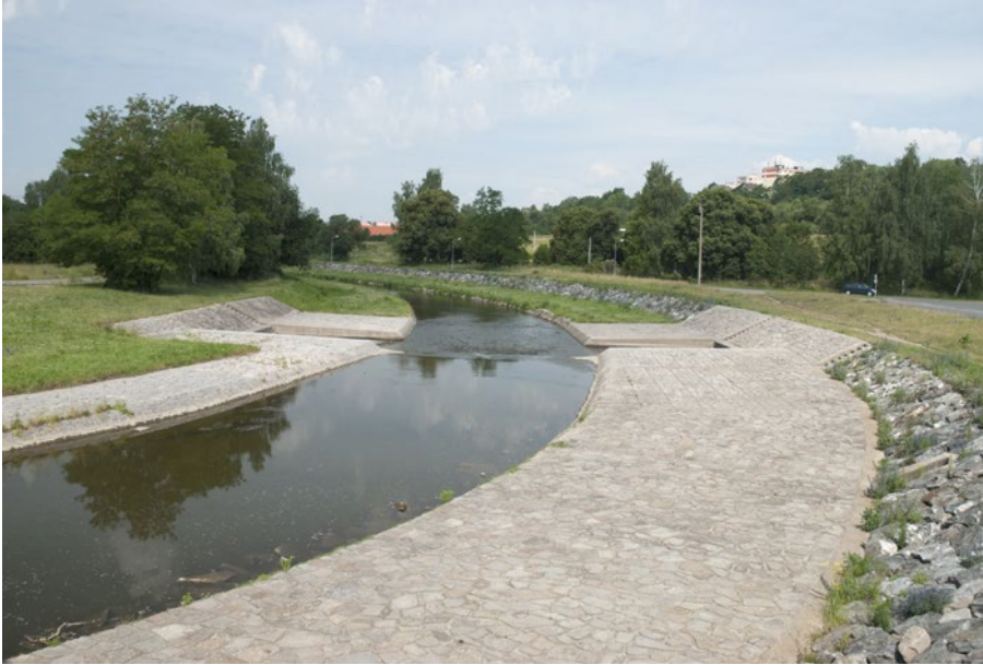
Fig. 93 Cuneette and berms of the stream channel, its fencing
