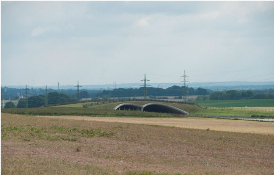
Fig. 119 Biocorridor on the bridge over the motorway = “ecobridge”
