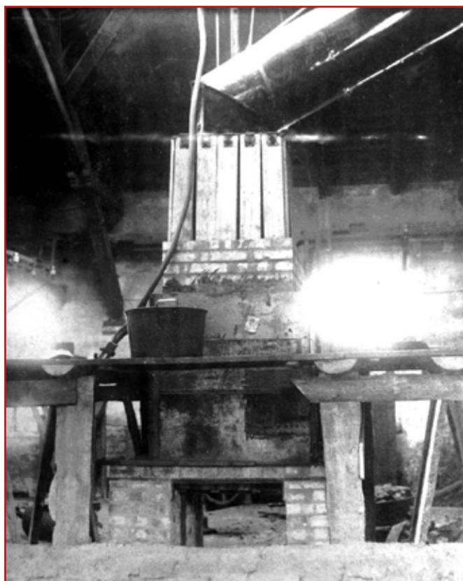
FIG. 3. *The first and oldest carborundum furnace in Benátky nad Jizerou (courtesy Carborundum Electrite a. s., Benátky nad Jizerou).*
