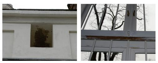
Fig. 1. Aesthetic defects: 1a - Left - incomplete facade surface, 1b - right - unfinished window frame coatings [1].
