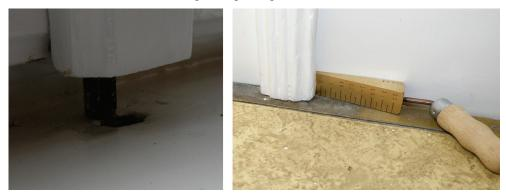
**Fig. 2.** Functional defect -2a - left - inoperative window fitting, 2b - right - large gap between the wings of the exterior door - measured by the measuring wedge - gap of approx. 6 mm, [1].
