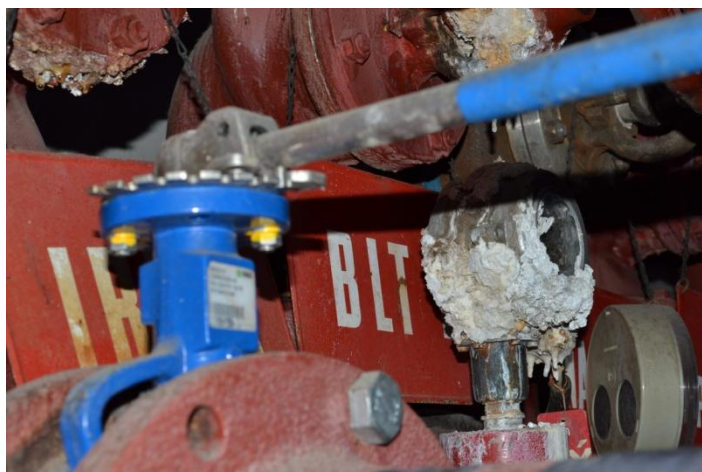
Picture 4.10. – Incrust on the surface of the relevant component at SLKP, a. s.
