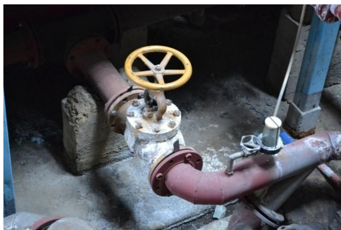
Picture 4.11. – Incrust on the surface of the valve at SLKP, a. s.
