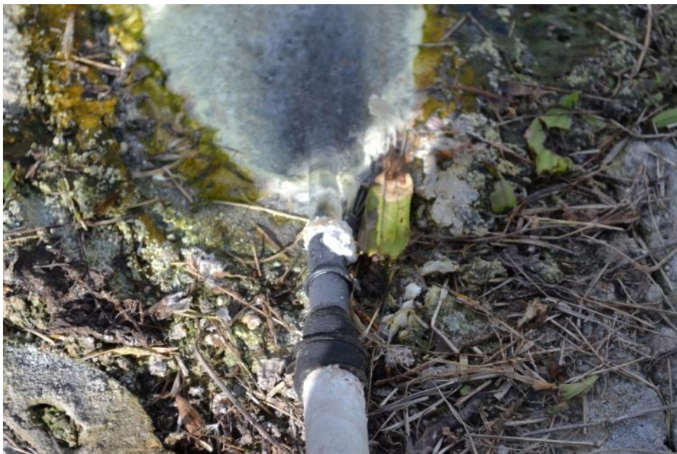
Picture 4.13. – Incrust creation around the supply pipe
